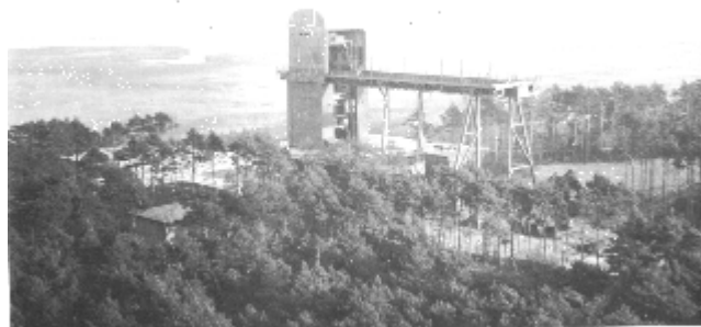
View of test stand No. 1 at Peenemünde A-4 engine and rocket propulsion test stand. Photograph courtesy of NASA-Marshall Space Flight Center
